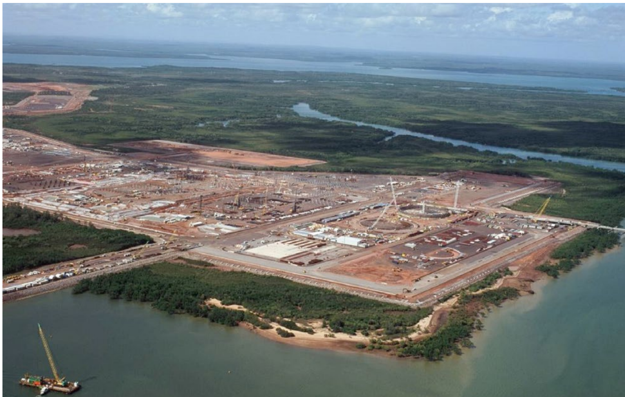
Aerial photograph of the Ichthys LNG plant near Darwin, Australia, early 2014
